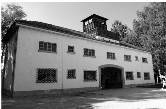
Dachau — Portão principal
